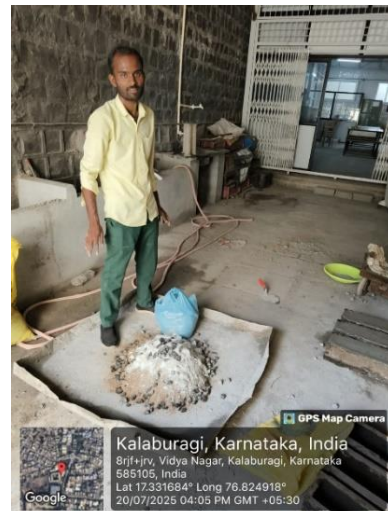
FIG NO.9 FIBRE CONCRETE MIXING
