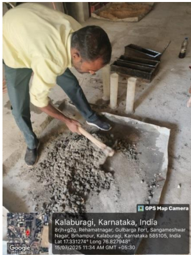
FIG NO.8 NORMAL CONCRETE MIXIN &
