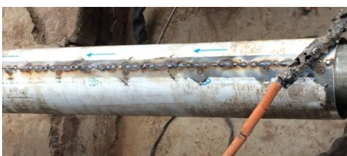
Fig. 5 TIG welding of cylindrical sheets
