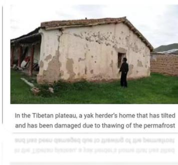
In the Tibetan plateau, a yak herder's home that has tilted and has been damaged due to thawing of the permafrost
