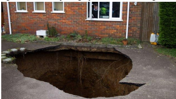
Fig. 1. Underground void near a house at Buckinghamshire, UK
