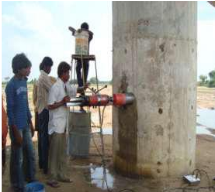
Fig 10 : Extraction of Concrete core from the Bridge Pier
