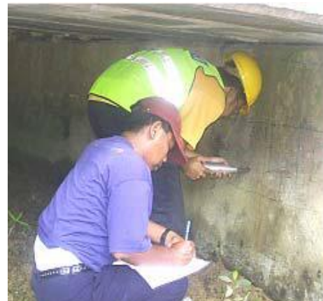
Fig 13: Rebound hammer test conducted on selected abutment
