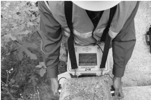
Fig 20: Application of ultrasound pulse velocity device on a concrete bridge wing wall.
