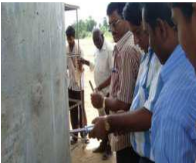
Fig 8 : Testing of Bridge Pier using Rebound Hammer
