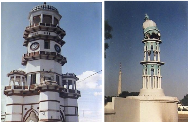
Fig 8 Damaged Clock Tower Fig 9 Mosque Tower at Sadar
