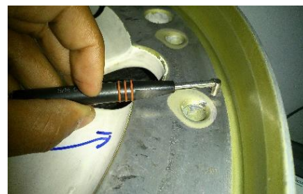
Figure: 4. Inspection around the bolt hole
