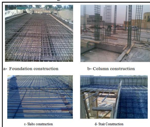
Figure 2: Different construction activities of building
